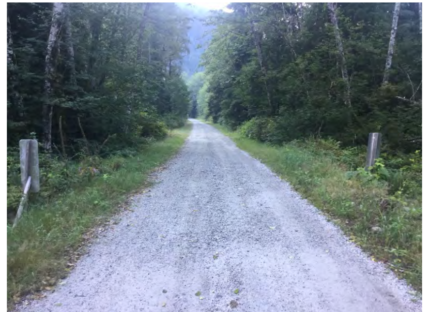
Left Approach Facing Away From Bridge
