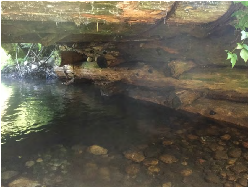
Left Abutment Note Slope of Logs
