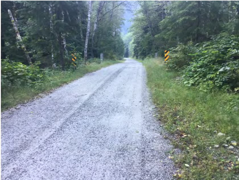
Right Approach Facing Bridge
