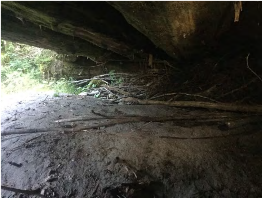
Right Bank Abutment
