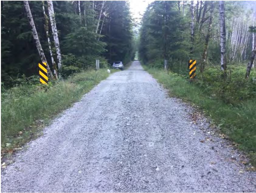
Left Approach Facing Bridge
