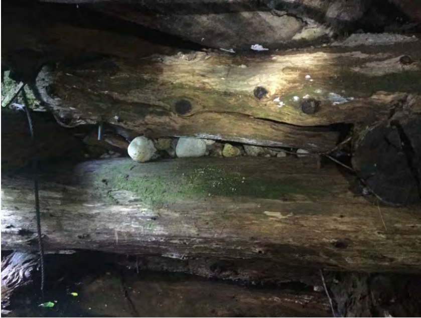
Left Abutment Split Crib Log
