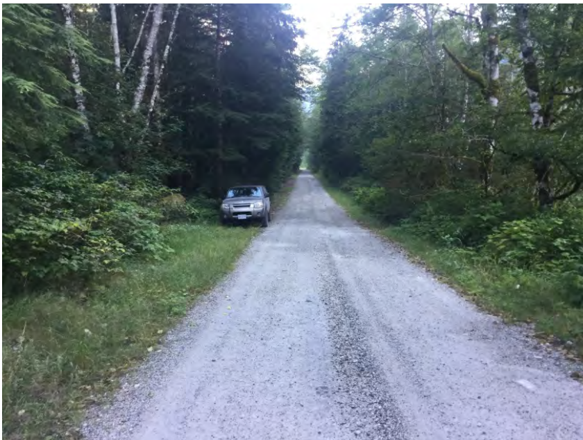
Right Approach Facing Away From Bridge
